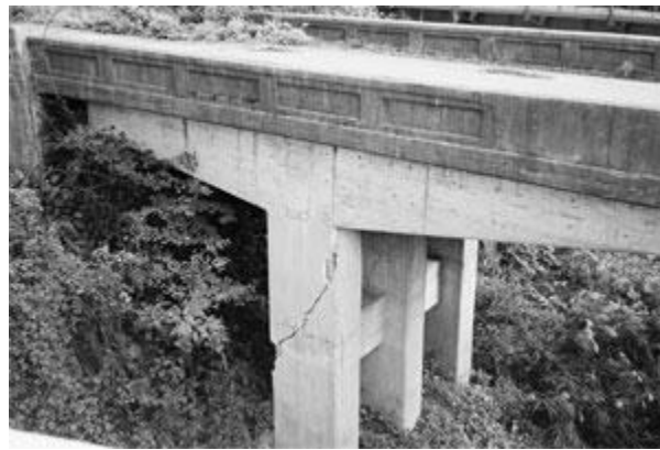
Columns of bridge
