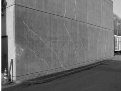
Figure 2.5. Thermal Cracks
