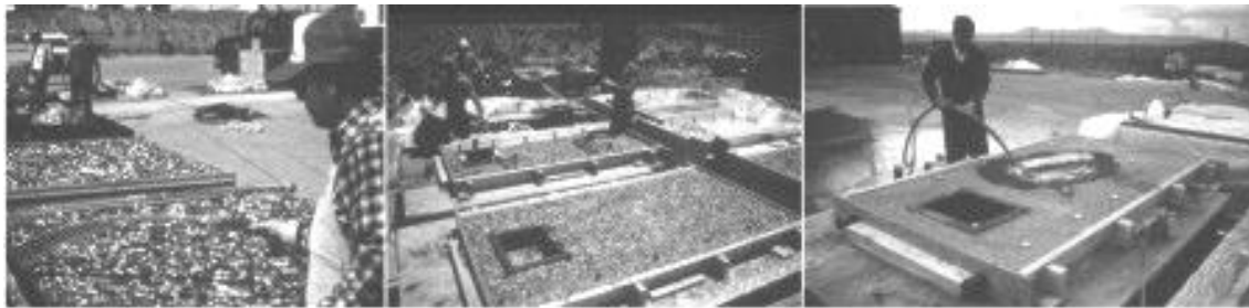
(i) Mould filled with fibres
