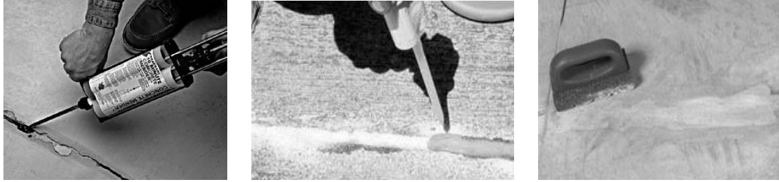
Figure 6.10. Epoxy concrete repair
