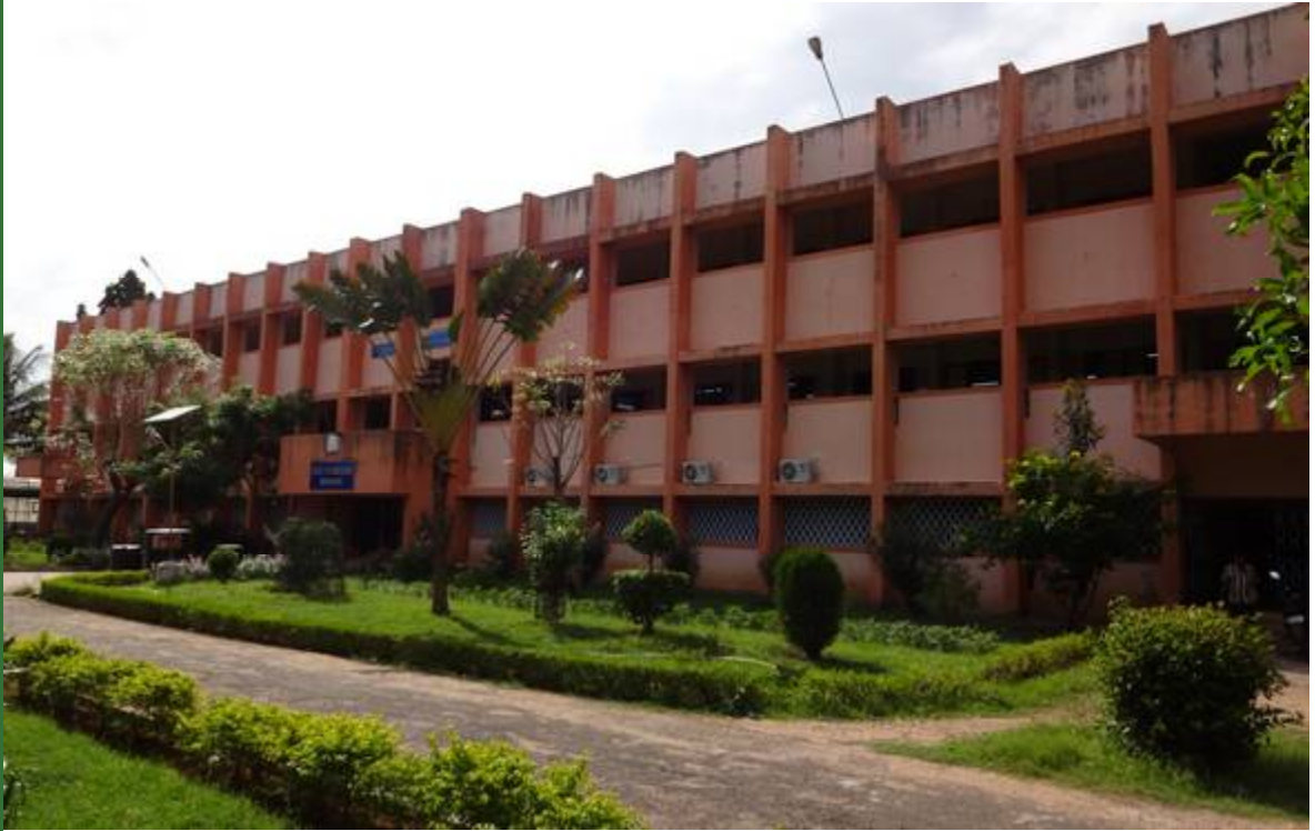
Class Rooms - New Block
