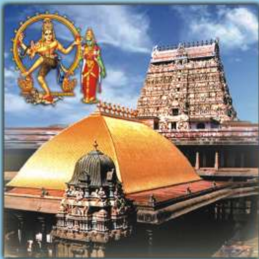
The Golden Roof at the Chidambaram Temple
