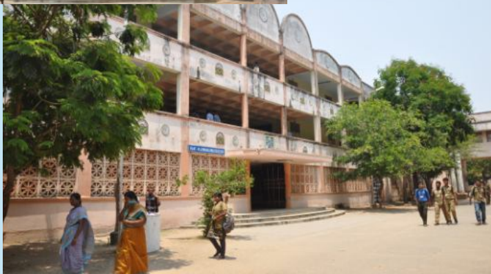
Class Rooms Platinum Jubilee Block
